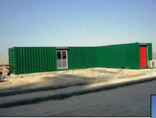
QC/QA requirements and need to have these on project locations, the mobile laboratory concept is quick and easy to install; these labs are not only configured with Tinius Olsen equipment but they can also accommodate equipment supplied by the End User on site. The novel use of retired shipping containers, rebranded by Tinius Olsen, is cost effective for our customers, supports efficient logistics and is environmentally friendly.
